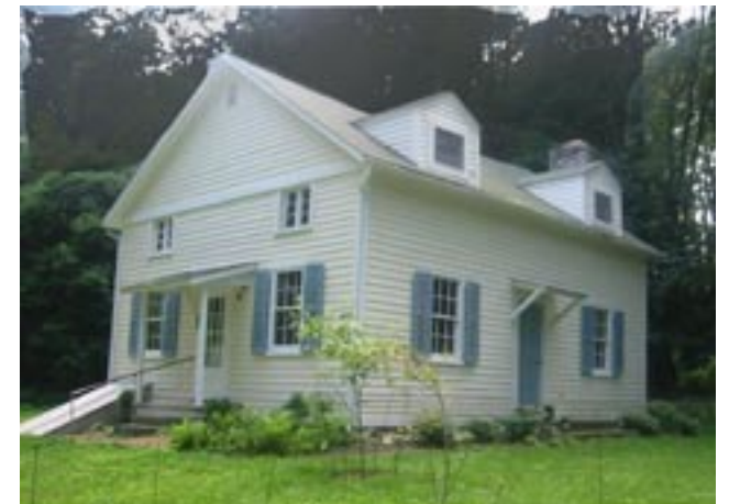
Cobb Road House Photo by Kitty Orth © 2004
